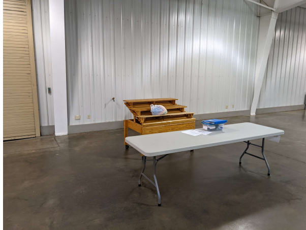
North wall, East of garage
