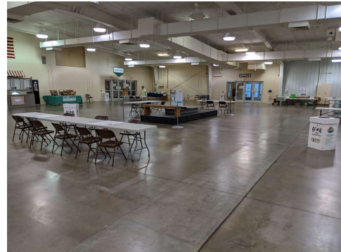
Facing SE corner
