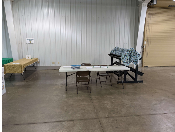
South wall, East of garage door
